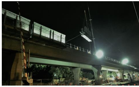
Supply of outriggers and permanent walkway steelwork
