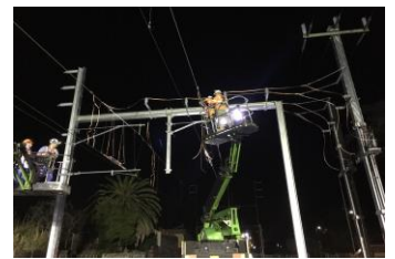
Supply of OHLE structures, Melbourne
