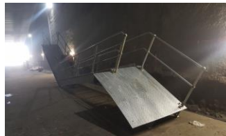
Westconnex staircase installation
