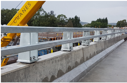
Albion Park Rail Pass
