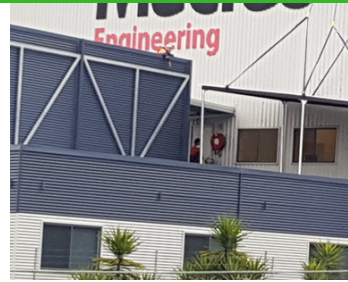
New smoko hut being lifted into place
