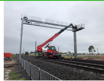
Albion Park Rail Pass
