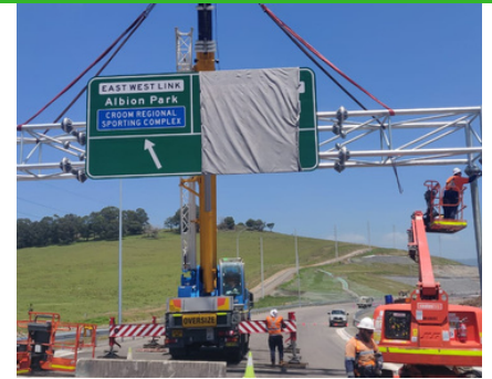
Albion Park Rail Bypass Sign Structures
