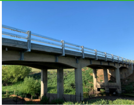
Install of posts at Demondrille Creek
