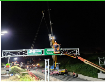
Albion Park Rail bypass sign structures
