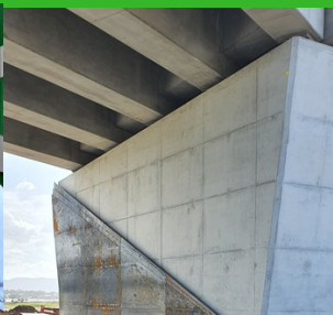
Core 10 wall Albion Park Rail
