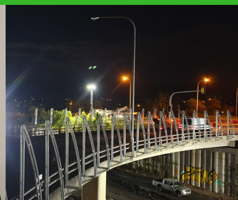
Albion Park Rail bypass sign structures (Oak Flats)
