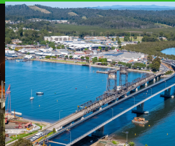
Aerial shot of Batemans Bay bridge (Courtesy John Holland)
